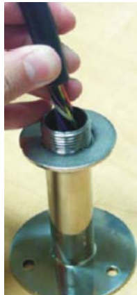
Figure 2-16: Running cable through the mounting pole
