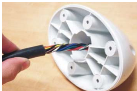
Figure 2-14: Running cable through the pole base
